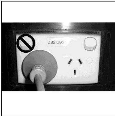
Ensure that the machine is switched off at the wall socket
